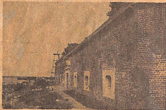
REMAINS OF ORIGINAL LEFT FLANK WALL
