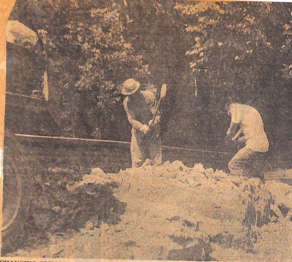
CHANGING BRIDGE — Above, workmen shown giving Stone Bridge a "face-lifting." Below is an earlier picture as the bridge then appeared, with pyramid in center and signs.
