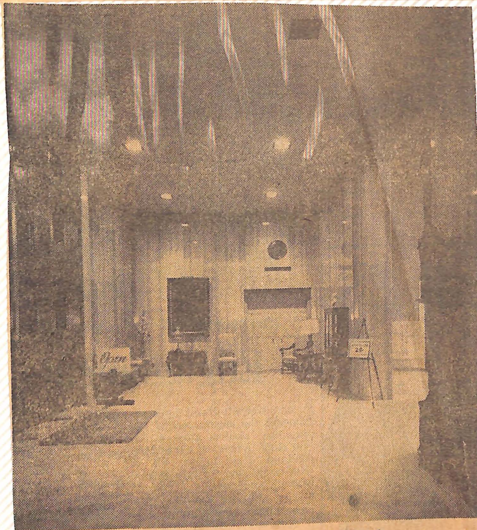
Entrance Hall Is Softly Lighted Handsome Bronze Doors Are on Left
