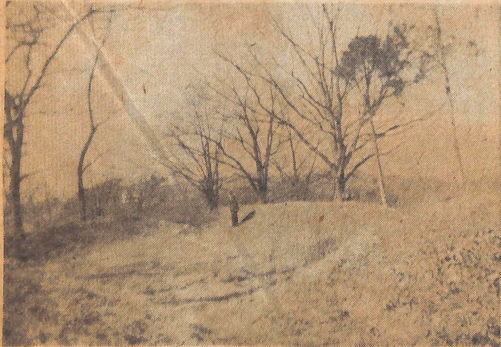
Confederates' Redoubt Above Rail Bridge Across New River
