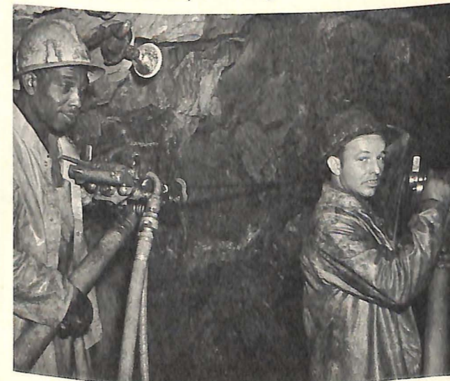
Work being carried on within the tunnel opening.
