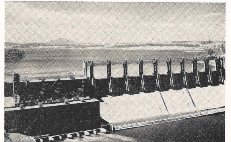
New River is dammed for the production of electricity by Claytor Dam of Appalachian Electric Power Company near Radford, Virginia. Claytor Dam has a capacity of 104,000 horsepower and is the largest hydro-electric development in Virginia and on the American Gas and Electric Company System.
