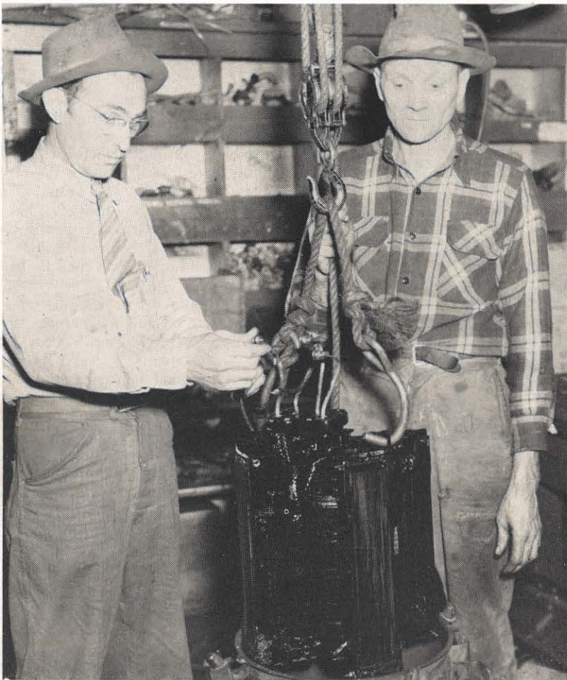
The substation department of the Pikeville district was kept busy last year. The employees of the department had 509 distribution transformers in their shop for checking and repairing. This was the largest number of transformers ever to be handled in the department in one year. In the photograph, M. C. Mutter, left, substation foreman, and Ireland Charles, maintenance man, give us an idea of some of the treatment the 509 transformers received in the shop.
