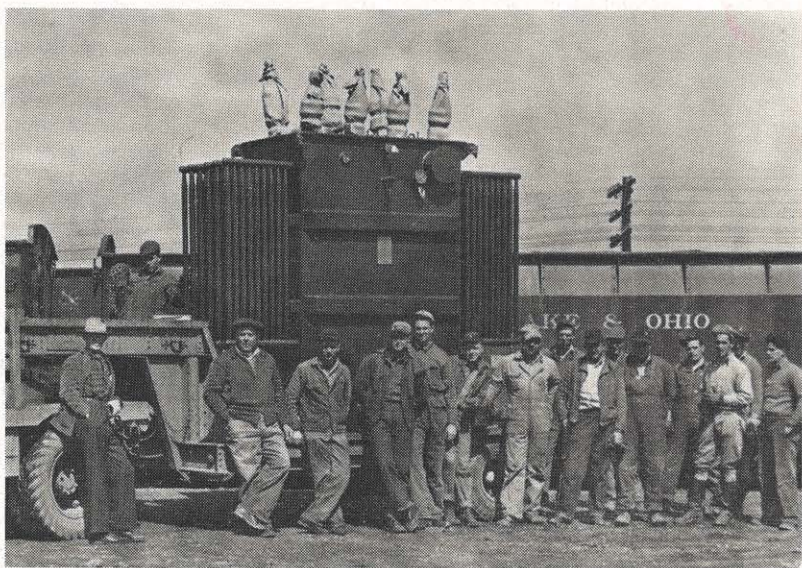
A Kentucky and West Virginia Power Company crew is dwarfed by the 10-ton transformer which is to be installed at a new substation near Louisa, Ky.
