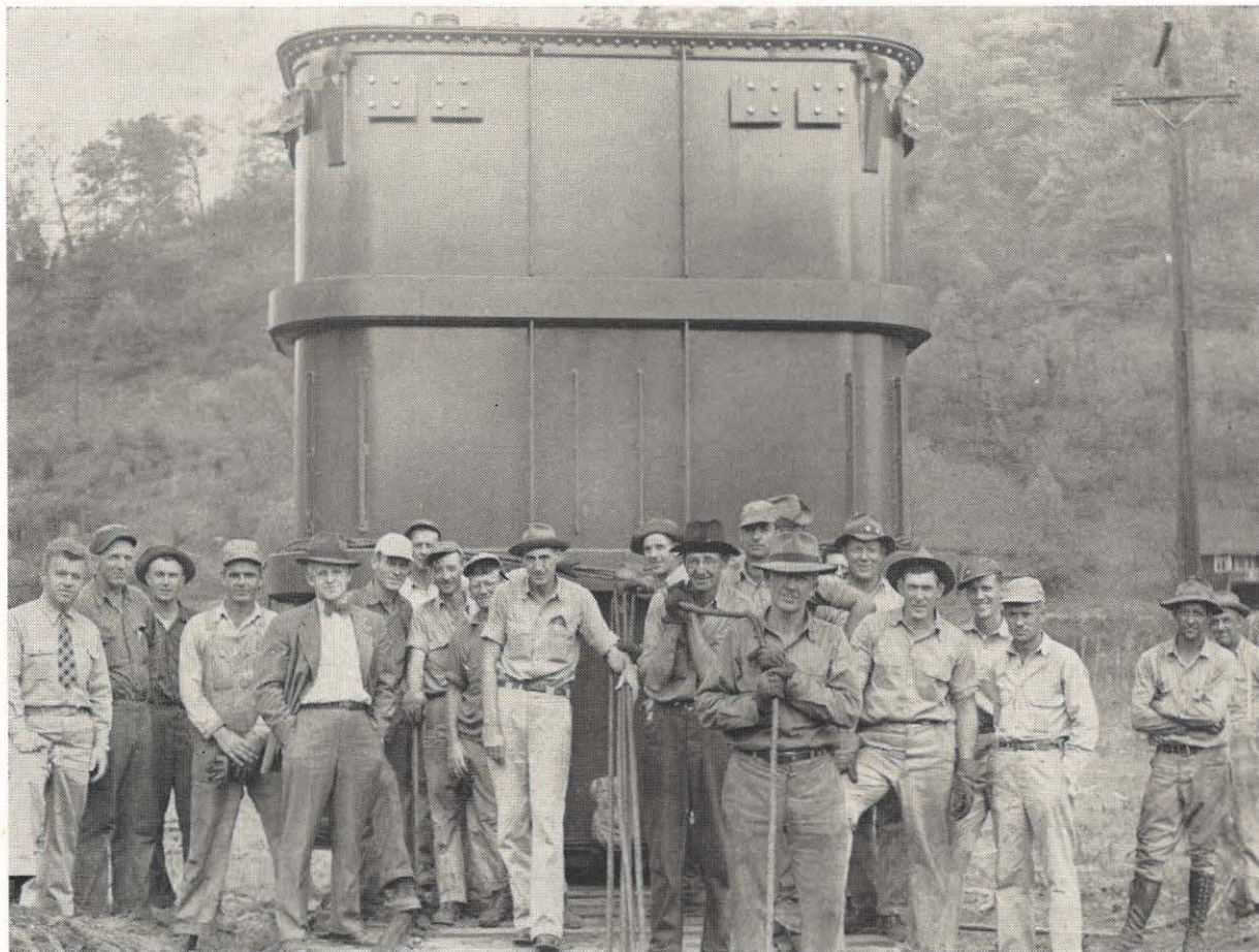
This 42-ton transformer is to be installed at the Betsy Layne, Ky., transmission station, which is now under construction in the Pikeville district. The men who were present when the transformer was moved from the flat car are, left to right: "Dutch" Rankin, system substation department; Albert Webb, Walter Billiter, Lee Compton, District manager F. M. Baker, Jess Mullins, Homer Helvey, Gratho Williams, Bill Harris, H. M. Eagle, Leonard King, Shirley Ratliff, Auburn Helvey, Jim Lowe, John Hunter, John Raine, Warnie Blackburn, Jesse Collier, Charles Stayton, Glen Whitt, Walter Smith and Ed Marrs.
