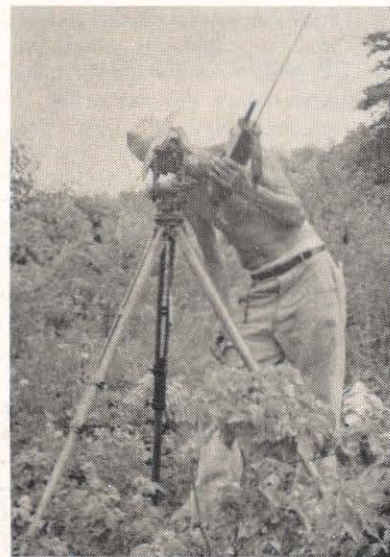
W. G. French, system transmission department, gives directions with "handie-talkie" radio during sagging operations.
