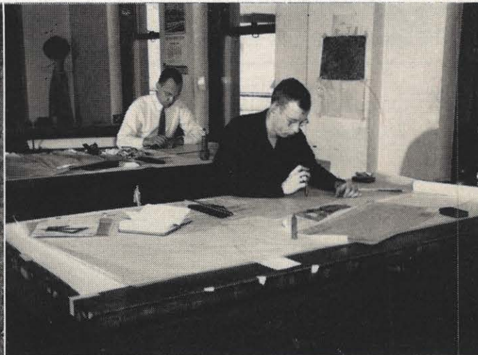
FINAL PLANS —After the survey is made and the right-of-way for the line is obtained, the final plans for the line are prepared. Draftsmen are shown above making complete drawings of the line, which show the number and exact location of the poles, and other necessary details.
