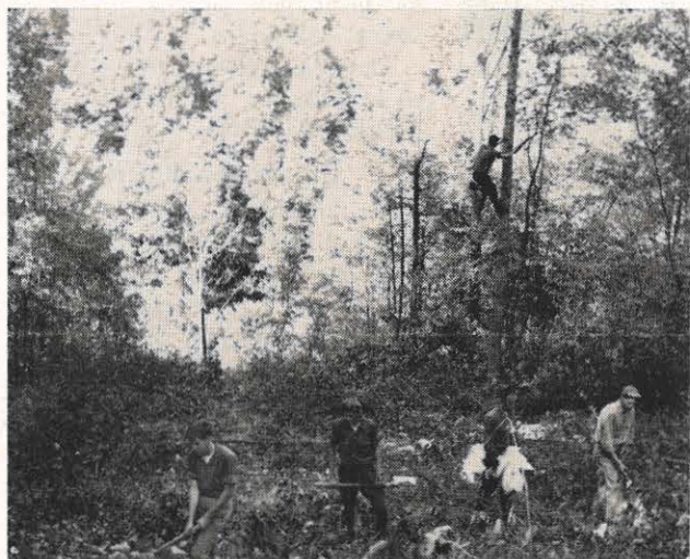
SURVEY CREW —After the information is received from the commercial department, studies are made by the technical section of the distribution department to determine the most practical route for the line. Then a survey crew, like the one shown above, is sent out to make the survey of the proposed line.
