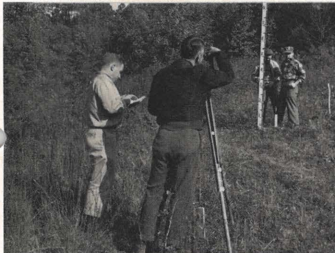
SURVEY CREW —After the information is received from the commercial department, studies are made by the technical section of the distribution department to determine the most practical route for the line. Then a survey crew, like the one shown above, is sent out to make the survey of the proposed line.
