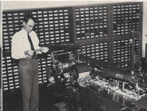
BILL PRINTING —The meter books are checked into the billing office and are worked on a prearranged schedule. Each ledger is readied for printing the bills. The machine shown here punches, perforates, prints, numbers, addresses, and cuts the bill, including the ledger sheet, to size. The individual postmark for each town is put on the bill along with the advertisement. Tom Barnett, operator of the printing machine, is checking a bill to see that the machine is functioning properly. The machine prints an average of 1,800 bills an hour.
