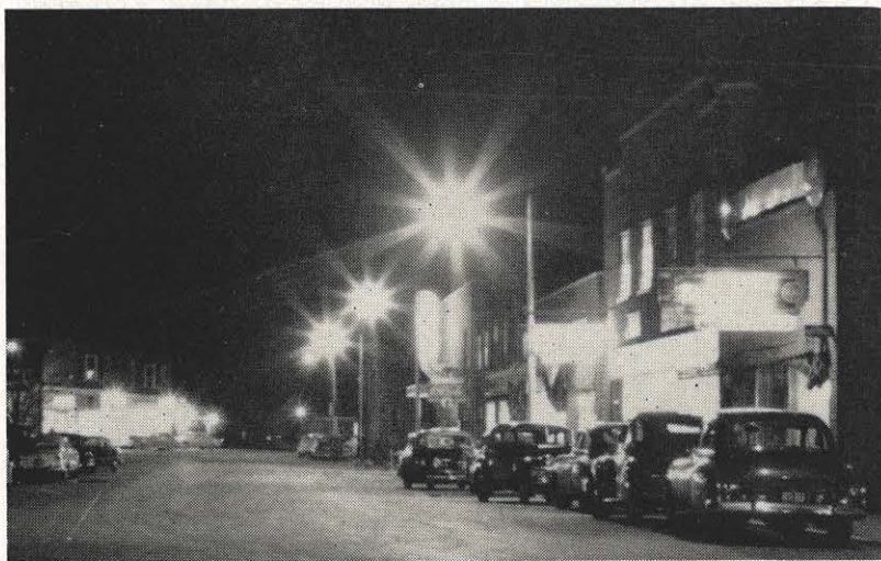
The Town of Saltville, Virginia, in the Pulaski district, recently had its street lighting system changed. Shown above is the new whiteway. The new street lighting is one of the major steps in a community improvement program which has been underway for the past several years. The new lighting system was installed by Johnny Sutphin, AEP foreman in the area, and his crew.
