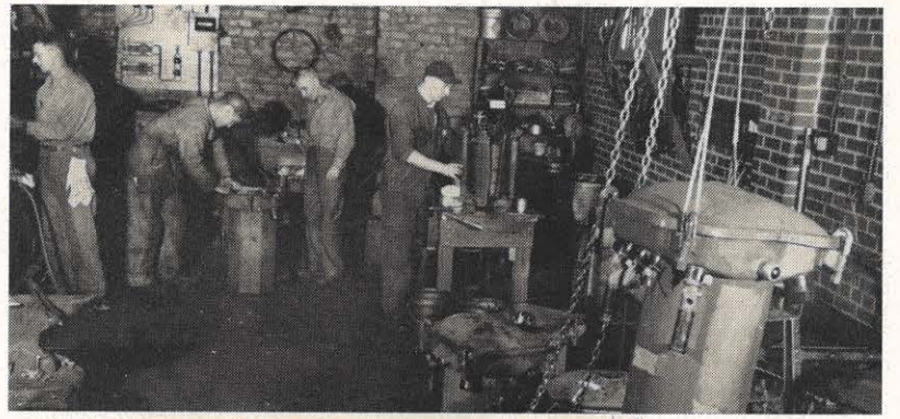
The Charleston district transformer shop made a record during 1950. The employees in the shop repaired, cleaned and tested 745 transformers during the year. Shown above in the shop are left to right: H. J. Spurlock, B. M. Harper, J. O. Bartlett and F. E. Porter.
