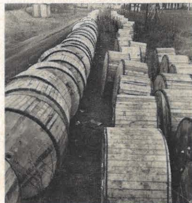
Reels of aluminum conductor are shown above at a roadside supply depot near Pratt, W. Va. These 3800-pound reels of wire will be used in the construction of the new double circuit 132 kv line from Cabin Creek to Glen Lyn. The double circuit line, connecting the two generating plants, will be erected by the way of Bradley and Hinton, W. Va. The interconnection is expected to be placed into operation by summer. Only a part of the reels are shown in this photograph.
