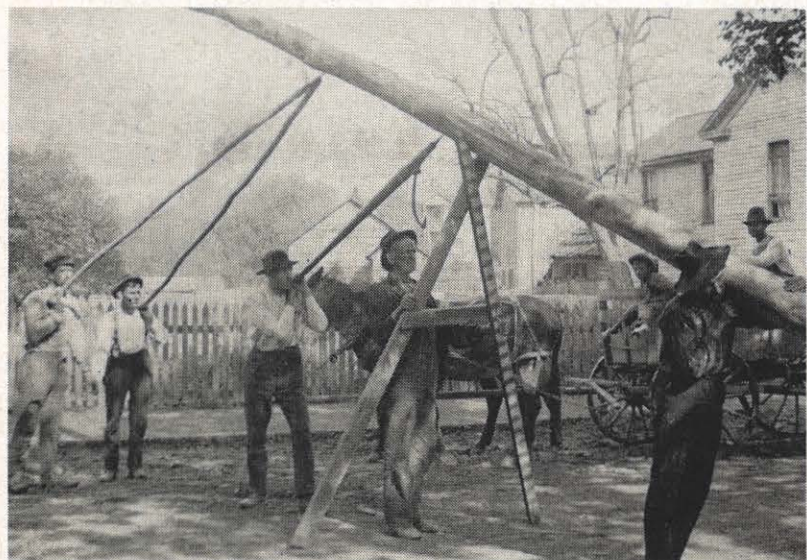
The picture above was made in 1905 and shows one of the first distribution poles set in Pikeville on Second Street near the corner of Division Street. Those in the picture who are identifiable are Milton Layne, young boy on the wagon, John M. Layne, shoulder under pole, and Benjamin Layne, holding the gin. They are the father, grandfather and great-grandfather of Milford Layne, stores department.
