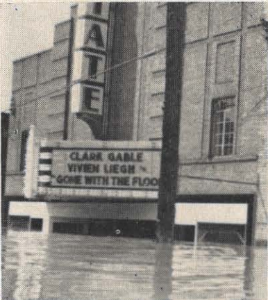
When the 1945 flood hit Point Pleasant, "Gone With the Wind" was playing at the State Theatre. As the water rose higher and higher, someone with a sense of humor changed the marquee sign to "Gone With the Flood." Residents termed this flood "mild, flood crest only 50 feet."
