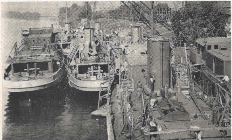
Men of the Marietta Manufacturing Company work busily to ready four more ships for service. This ship building yard above Point Pleasant is the only one of its kind on the Appalachian system. In the background are ships under construction, being made ready for launching by sliding sideways down rails into the Ohio River.
