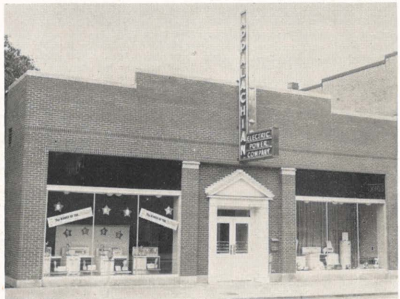
Abingdon District Office Building
