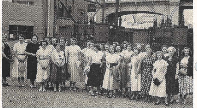
Members of the Bluefield Girls' Service Club visit one of the company's substations while on tour of some of the company property.
