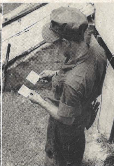
Bill checks the tags from the meter and the jumper to make sure he has the right meter at the Casto home. The tags are returned to the laboratory and checked with a third section which has been held as a receipt.
