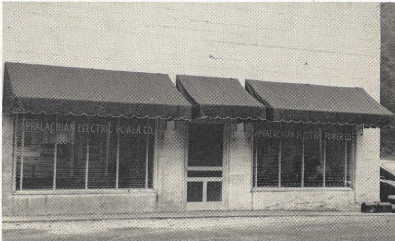
A new Logan district office at Man, W. Va., shown above, was formally opened to the public Saturday, July 21. The new quarters, established to serve area customers, is equipped with a large business office, community room and a demonstration kitchen. The new office will be staffed by Paul Jeffrey, area representative; Martha Booth, home economist; A. M. Payton, local representative; Dawna J. Perry, cashier, and Dorothy Browne, maid.
