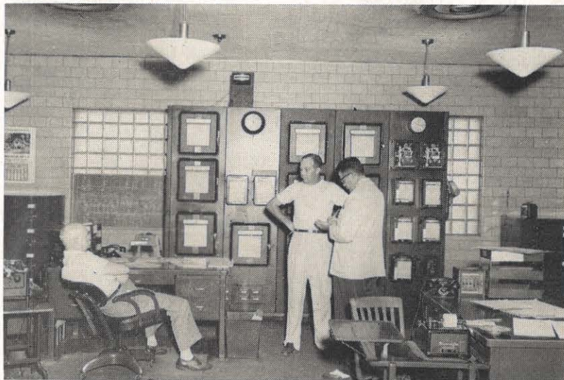
C. L. Vest, seated, and F. H. Rouse tell W. R. Witzel what they were doing when lightning struck an alcohol tank at the near-by Institute plant of Carbide and Carbon. The explosion knocked down the two lights in the foreground, the one on the left hit the floor at the edge of the chair mat while the other fell on top of the desk.
