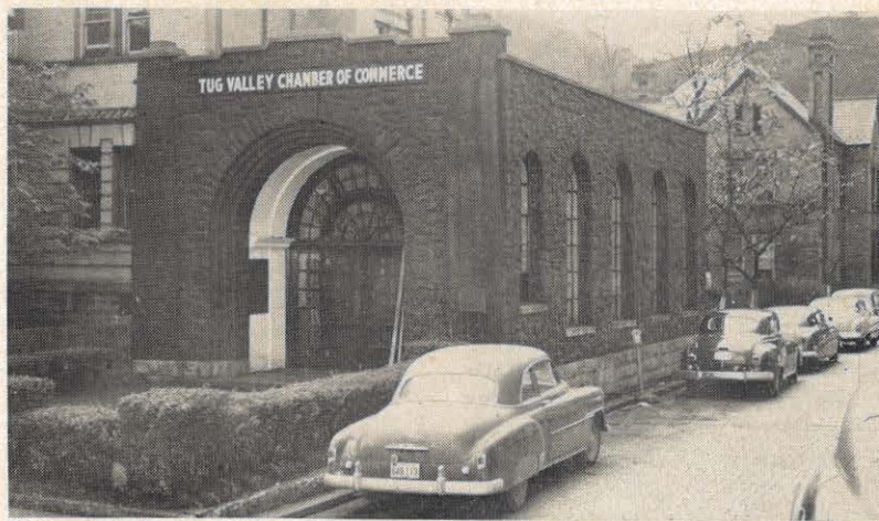
Built of coal in 1933 from the famous Winifred seam, the "Coal House" is one of the most unusual buildings in the nation. About 65 tons of coal were cut to fit as building stone. Varnish is applied periodically to prevent wearing away caused by the weather. This building in the business section houses the Chamber of Commerce, the Junior Chamber, the Credit Bureau and the Area Boy Scout Executive.
