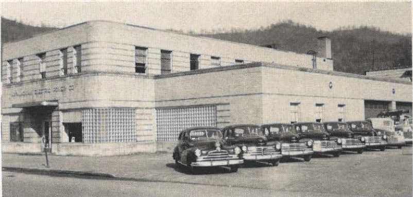
Headquarters for the district serving parts of seven counties in West Virginia and Kentucky is the Williamson district office building. Here T. M. Watkins, district manager, directs the activities of 120 employees who serve almost 20,000 customers with about 1,200 miles of line.
