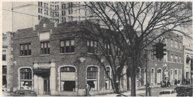
The Kentucky and West Virginia Power Company office in Ashland serves as headquarters for the company and the district. R. E. Doyle, Jr., general manager, and H. S. Scott, assistant general manager, direct the activities of the company's employees. The 177 Ashland district employees serve over 26,000 customers in parts of the counties of Boyd, Greenup, Carter, Lawrence, Rowan, Elliott and Lewis. Behind the office towers the Second National Bank.
