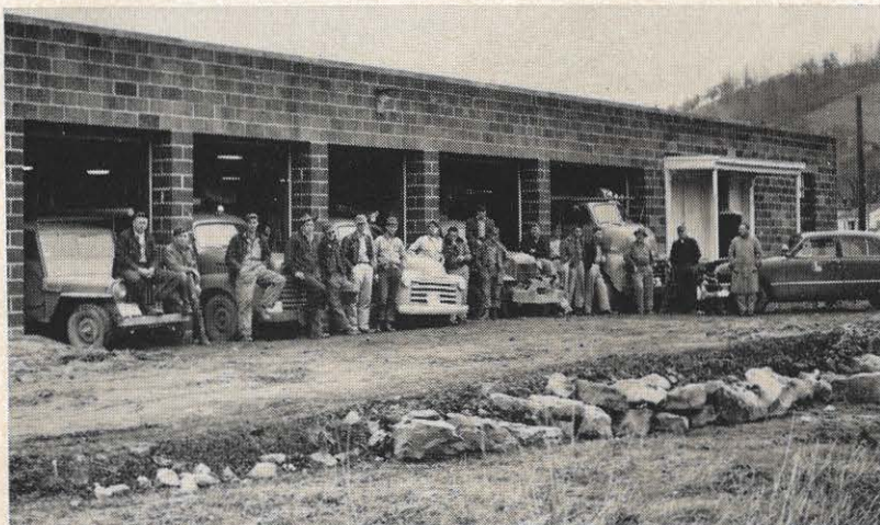
Lined up in front of the new Clintwood service building are members of the Abingdon district transmission and distribution department. From left to right, are: J. A. Self, S. S. Stevenson, R. C. Childress, J. A. Arrington, L. R. Vaughan, W. H. Coe, J. S. Barrett, C. E. Rosenbalm, R. A. Shaffner, I. H. Mace, C. M. Jackson, C. W. Hale, E. L. Rasnake, W. L. Smythers, C. J. Miller, J. S. Mize, C. C. Self and W. H. Ferguson, rural department. The building is 45 by 90 feet and provides storage space for materials and vehicles as well as housing office space for the foreman, timekeeper and serviceman.
