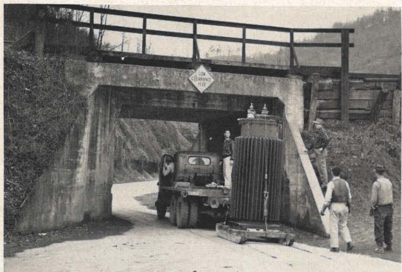
It was a close fit to get the 500 kva transformers for Jackson substation in the Hazard district under the bridge pictured above. Loading each transformer on a sled, it cleared the underpass by inches after the primary bushings were removed. Pictured above are: Robert Adams, driving truck; James Burdsal, rear end of truck; Gaine Stidham, standing on bank; Ernest Pennington and Hayes Stidham, walking behind the transformer.
