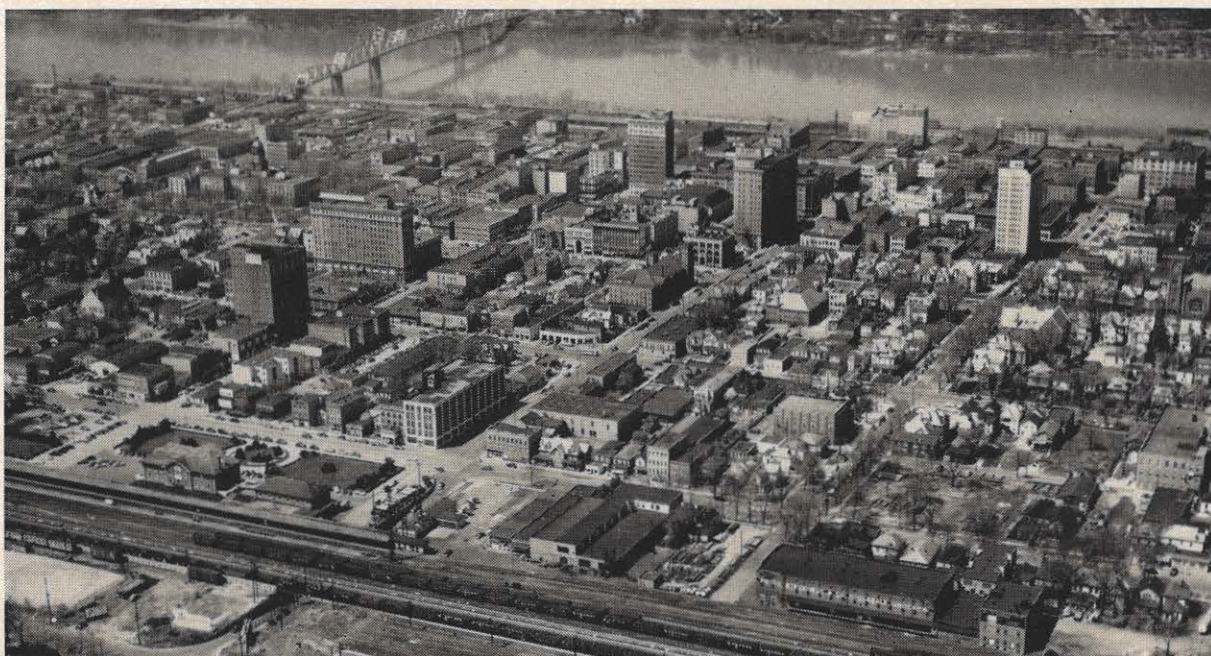
Huntington's skyline rises sharply from the edge of the Ohio River. This aerial photo shows the city's business section from Seventh to Eleventh streets, left to right, and from Second to Eighth avenues, top to bottom. Credit for planning the city's wide streets and avenues goes to Rufus
