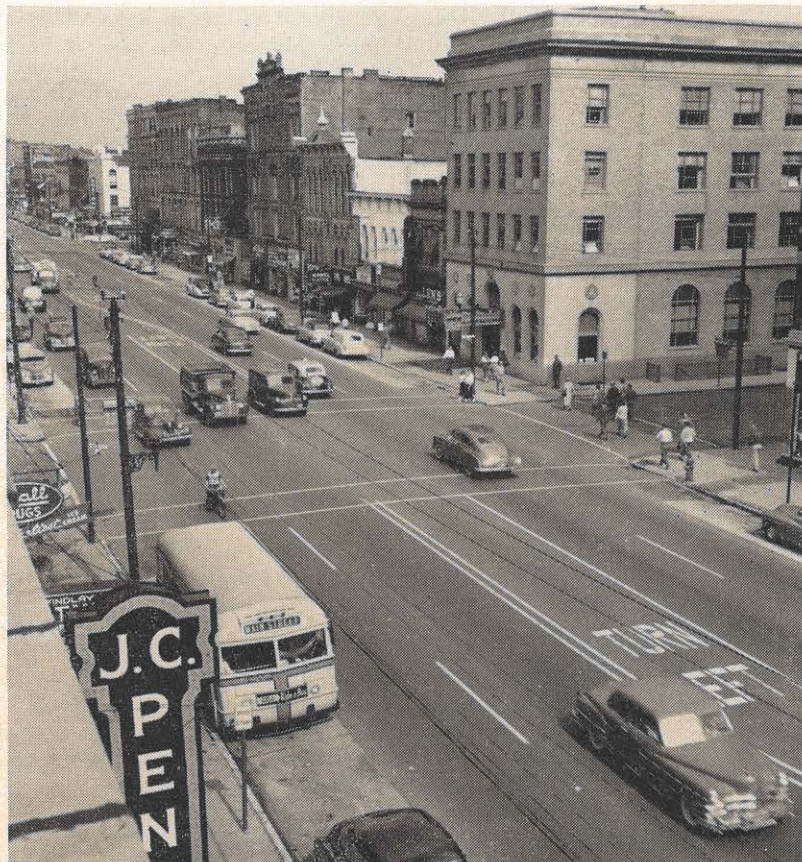
Looking north on Main Street in Findlay, Ohio, headquarters of the Central Ohio Light and Power Company which last year became a part of the A. G. & E. System. Central Ohio serves over 23,130 customers and 46 communities.
