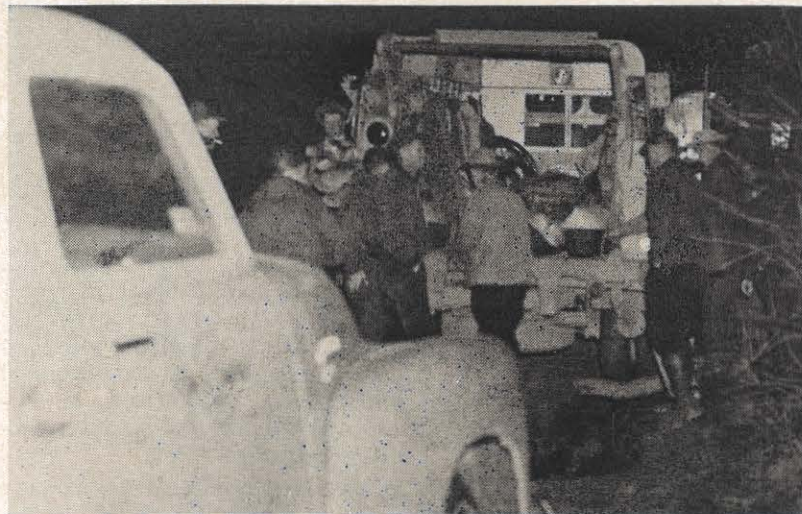
It's still dark when the Pikeville district men arrive at Gibson substation and prepare to unload tools and equipment.
