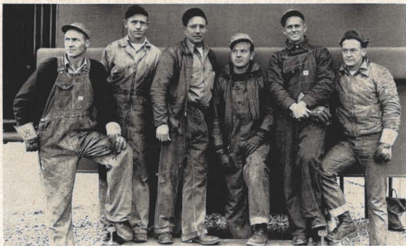
Members of this hot-line crew of the system transmission line department at Bluefield recently completed an unusual job for the Ordnance Plant of the Holston Defense Corporation at Kingsport. The job required the replacement of defective bus connections, switch cross arm supports and one 50-foot pole in a six-pole switching structure. All the work was done without interrupting the 132,000-volt service. Left to right, above, are: K. A. Hayes, F. T. Combs, J. B. Doss, foreman, who planned and supervised the work, C. H. Hager, C. W. Edmonds and S. N. Burchette.
