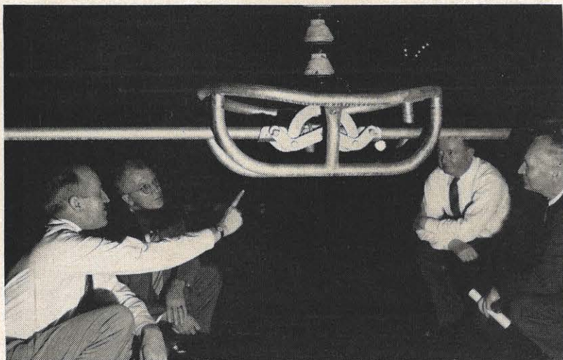
R. L. McCoy, of Locke Insulator Corporation, shows a 500,000-volt insulator shield and conductor clamp to I. W. Gross, E. L. Peterson and F. A. Lane, three AGE men in the research program.
