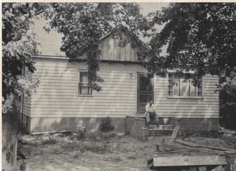
George Jeffers takes time out from his house-building duties long enough to sit in front of his new home which is nearing completion.
