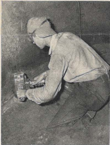
Okey Bailey grinds the welds to finish the job.
