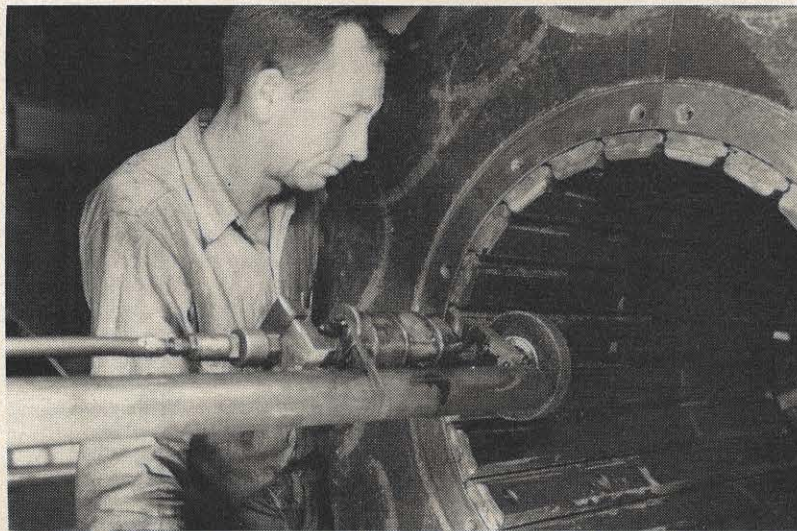
L. H. Carnifax, maintenance mechanic, sets up the cutting operation on the London hydro shaft bearing at the Cabin Creek plant. The bearing surface was ground within .003 of an inch of the actual drive shaft diameter.
