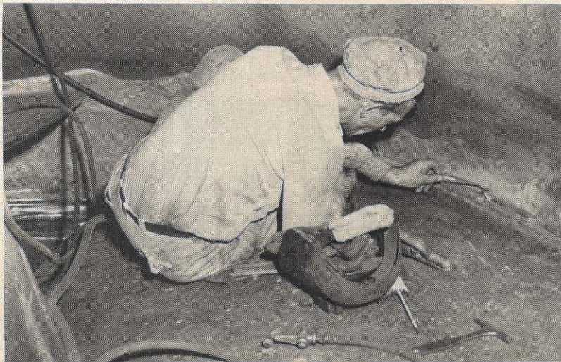
C. C. Jackson inspects a weld on the edge of a blade.
