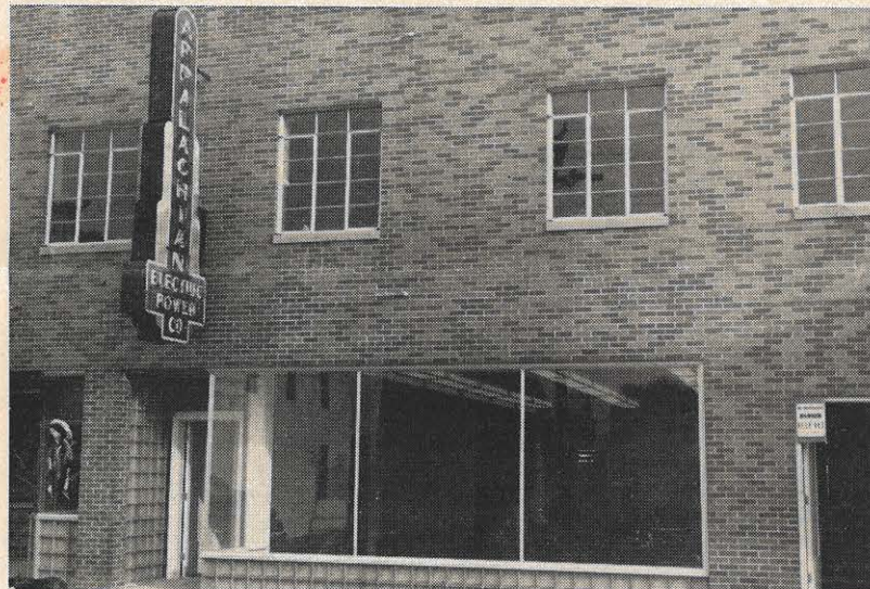
The new Oak Hill office is shown shortly after completion in October
