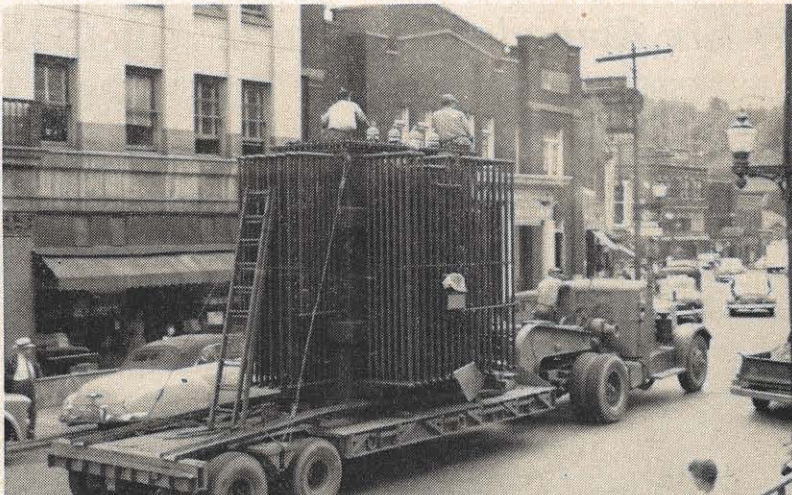
This giant 6,000 kva transformer was being moved through the City of Bluefield by J. D. Wingfield's substation maintenance crew when the above photo was taken. The transformer, for the South Bluefield substation, contains 3,000 gallons of oil and is the third such unit to be installed at the station.
