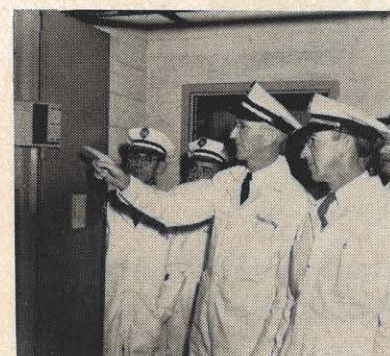
J. J. Roseberry, Abingdon district line foreman pointing to the electric panel board, recently was named chairman of the Johnston Memorial Hospital evacuation committee at Abingdon. Roseberry is describing switching arrangements of the 10 kilowatt portable generator to members of his committee. The rescue group will work out detailed plans for safely removing patients from the hospital during emergencies. The committee is composed of outstanding members of the Washington County Life Saving Crew.
