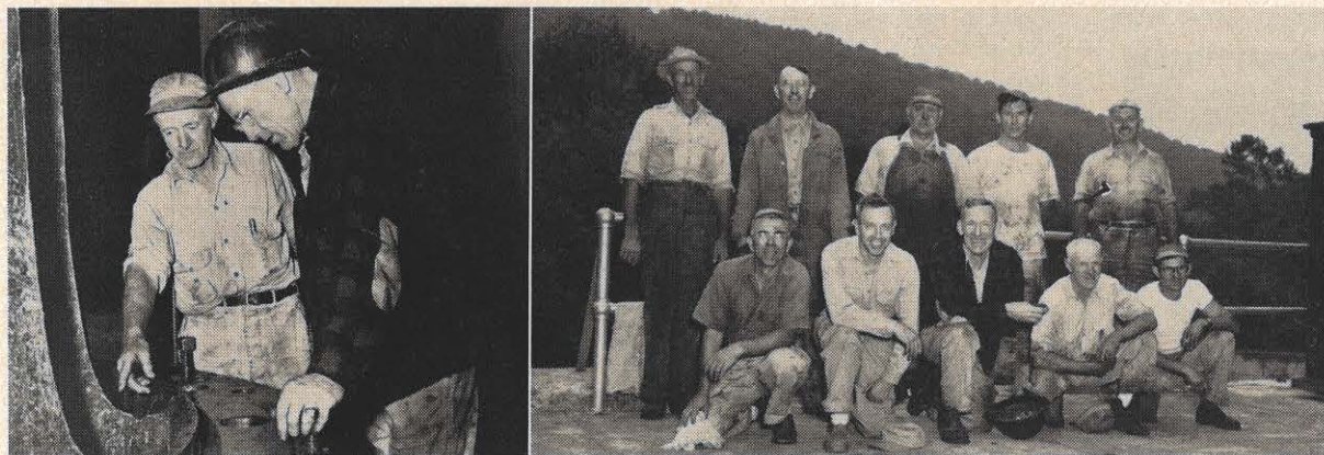
LEFT: Foreman Mustard points out damage done to turbine bucket by erosion and cavitation to Supt. Clark. RIGHT: The maintenance crew is pictured after a day's work. Kneeling from left: Cabbie Littreal, Frank Bargar, Red Clark, King Mustard, and Walter Taylor. Standing: Hurley Rotenberry, John Dent Burnette, Eathel Porterfield, Earl Shaw, Jr., and Otey Rhudy.
