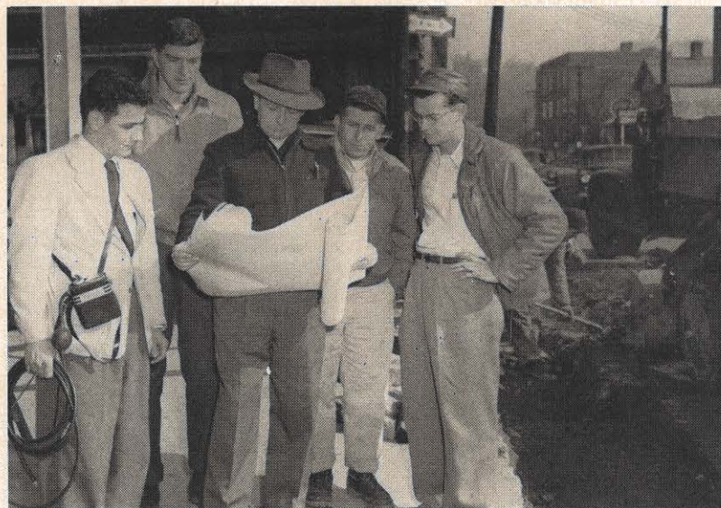
These Charleston employees are busy supervising the work of putting the lines underground in the downtown area of West Virginia's Capital City. From the left are: Paul Skaff, John Bailey, Don Newman, Cam Coffman and Ken Judy, Jr.
