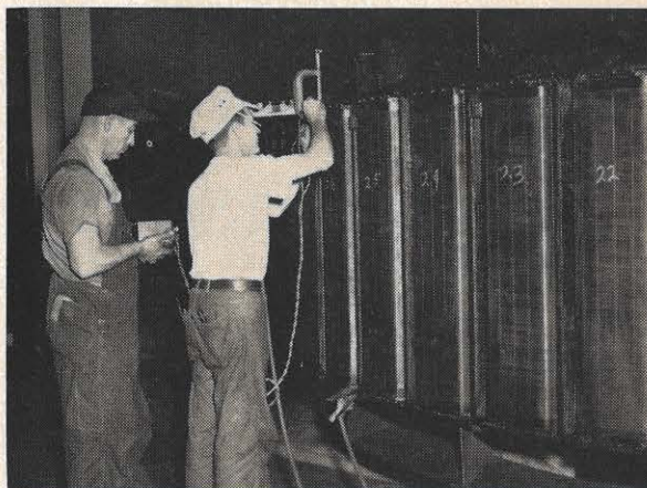
Left, company employees complete one of their final inspections before assembly by checking electrical connections on the damper winding in the 90-ton generator field while the shaft is out. Right, members of the crew completing this maintenance project, left to right, front row, are: A. D. Thornton, W. H. Brodie, Jack Davis, E. E.
