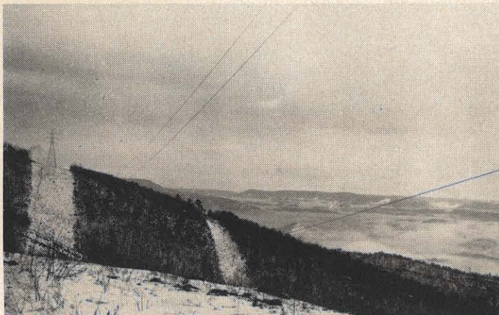
Left, a view from the base of tower twenty-two shows the dense haze hovering in the valley below. Right, general foreman Roy Doss inspects the damage to the conductor and the insulator.
