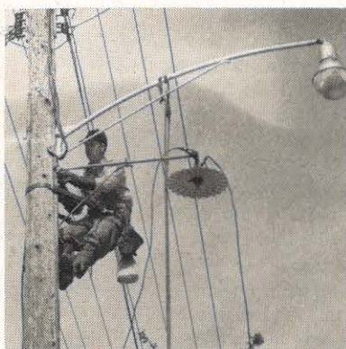
L. A. Philpott, lineman at Rocky Mount, removes the old street light fixture after connecting the new.
