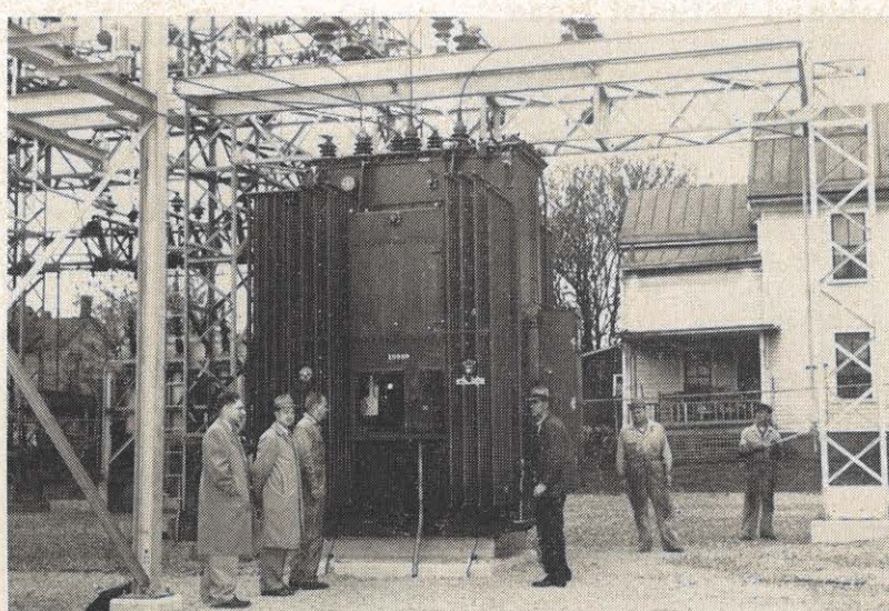
This new 5,000 KVA transformer recently was placed into service at the Seventh Street Station in Roanoke. This additional capacity raises the total to 20,000 KVA serving the underground distribution system in the downtown section of the city. The network has been served from thirty underground vaults of variable sizes. Construction is currently underway on four new vaults and the increasing of the size of three existing ones. Looking at the transformer is put in service are, from the left: D. D. Neilsen, General Electric Company; R. A. Armistead, W. S. Jones, W. S. Shanks, R. G. Amos, Jr. and R. W. Swain, all of the Roanoke Substation Department.
