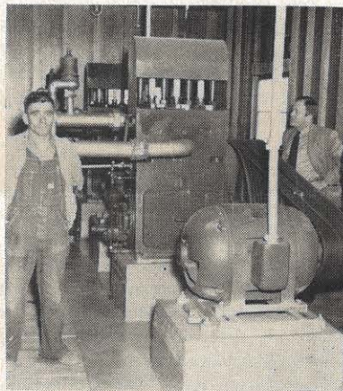
Jarrett Wood, Pikeville district engineer at right, looks over one of the water pumping stations which has two 50 hp pressure pumps for water injection.
