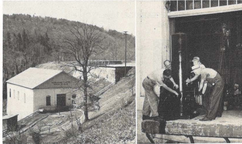
Left, Appalachian's Niagara Hydro Plant. The intakes at the end of the canal can be seen above the plant while the river winds below. Right, Niagara personnel slide a governor oil pump and tank to the ramp as dismantling begins.
