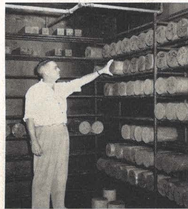
Inspecting a concrete cylinder sample in the lab curing room near the Philip Sporn plant is H. P. Hatch, AGE engineer in charge of concrete work.
