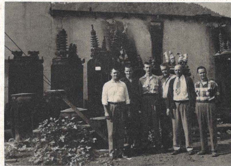
Helping check the fire which threatened these transformers beside the Guyan Inn were, from the left: Homer W. Dyer, Alvie Napier, Donald R. Coffey, Woodrow W. Dalley, Warren C. Workman and Lovell McDonald. Others who helped were Oscar Thompson, John Jones, Walter Blankenship, Dallas Hayner, J. S. McNeely, Carl Parsons and E. L. Kimmell.
