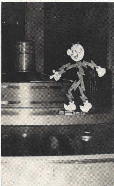
Reddy is a hydro man, too. He inspects the units at Claytor Hydro Plant while touring the Pulaski district.
