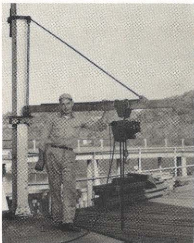
Clarence rigs the finished product on an I-beam to demonstrate its operation. He was assisted in making the boom by three men in his crew.
