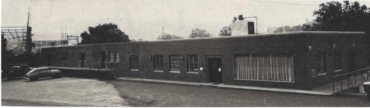
The new addition to the Fieldale office building is on the right, measuring 60 by 45 feet.
