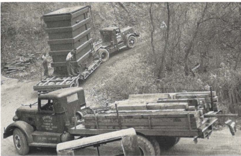
This turn was one of the difficulties in moving the new 10,000 kva transformer to the Leslie County station in the Hazard district. Weight of the transformer when assembled is 125,000 pounds. This unit was received at Yerkes, Kentucky, and moved to Leslie station under the supervision of the system substation department. This makes the second 10,000 kva unit installed at the station. The new unit is expected to be put in service next month after work is completed by personnel of the Hazard district and the system substation department.
