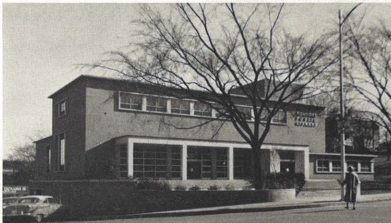
The modern Roanoke Public Library building is one of four in Roanoke with a commercial heat pump installation. The heat pump in the library like most commercial pumps is tailor-made.
