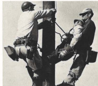
Following pole top resuscitation, the victim is made ready for lowering to the ground. Radford powder plant linemen C. W. Asbury and M. E. Morris work with Jack Kidd, Pulaski district lineman who is the victim.
