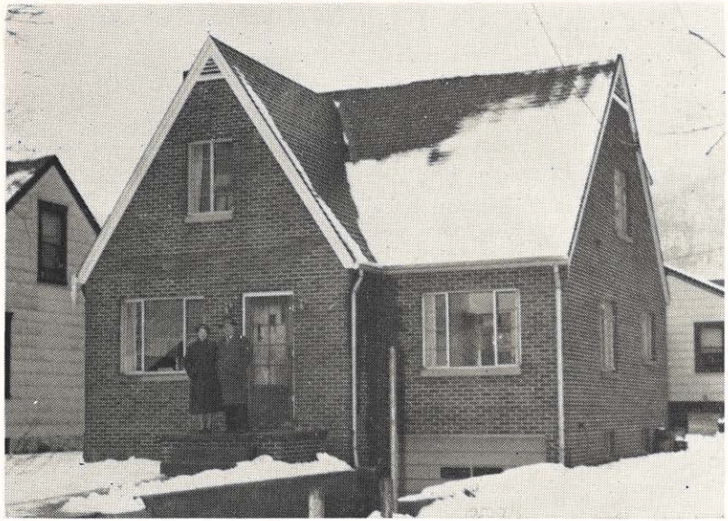
Mr. and Mrs. J. M. Kauffman stand proudly before the home which he built at night and on week-ends. Notice the basement garage at the lower right and the frame house he built 20 years ago on the right edge of the picture.
