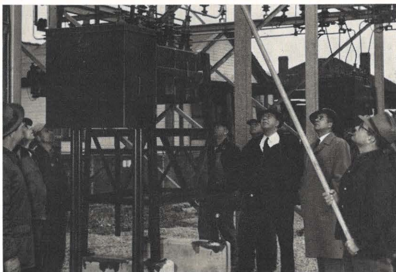
A 12,000-volt switch is closed by A. J. Wilkinson, general serviceman, as a part of the energizing of the first section of the company's underground power distribution system to downtown Charleston. Looking on when the switch was closed were C. M. Shafer, M. A. Myers, Steve Didier, W. E. Lacy, Charles Kelley, R. H. Hayes, L. M. McKibbin, W. R. Witzel and George Hervey. (Photo courtesy "The Charleston Gazette.")
