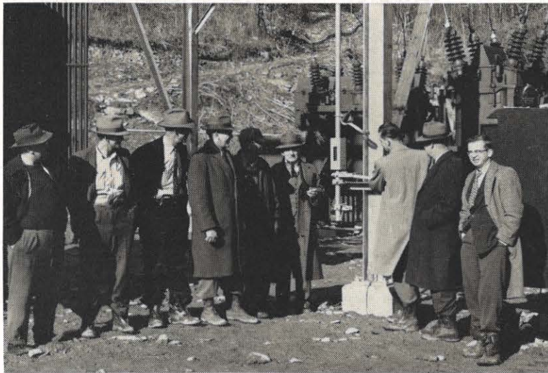
A new substation, known as the McDowell Station, at Bishop, Virginia, has been put in service. The 7,500 kva capacity station provides an additional source of power to the Bishop-Faraday area in the Welch district. Shown throwing the switch is Marvin Bostian of the Bluefield division engineering department. From the left in the photo are: G. E. Adams, Ralph Slade, J. D. Dalton, C. R. Settle and J. W. House, all of the Welch district; A. L. Wellford, Mr. Bostian, Paul Hilliard and Harry Garber, all of the Bluefield division engineering department.
