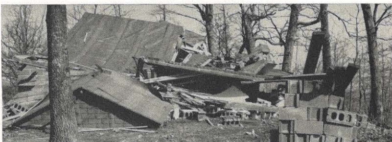
This was all that was left after lightning hit a tree and caused the collapse of the Mt. Zion Baptist Church atop Crumpler Mountain in the Welch district. At the base of the tree about 25 feet from the building there were several large holes showing the path of the lightning before it hit the end of the building. The meter on the church was completely destroyed; parts of it were found 30 feet away. The bolt also destroyed another meter 300 feet from the church and a fuse cutout eight spans away from the church, causing an interruption to about 20 rural customers. A 3 kva transformer fuse a mile away was also blown. An old-timer in the area said it was the most terrific bolt of lightning he had ever seen.
