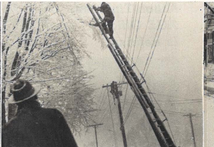
Huntington linemen went to work under difficult conditions to clear the trouble. Here Edward Stump removes a limb from the wires.
