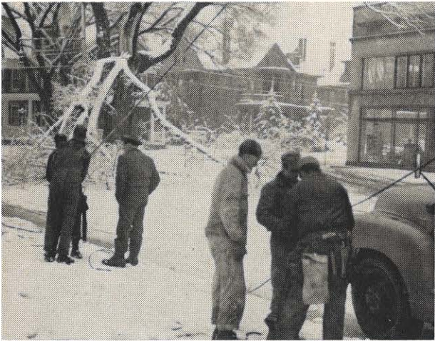
Charleston was truly snowed under with lines down everywhere. C. M. Shafer's crew is shown on Brooks Street re-stringing lines broken by that giant tree limb.
