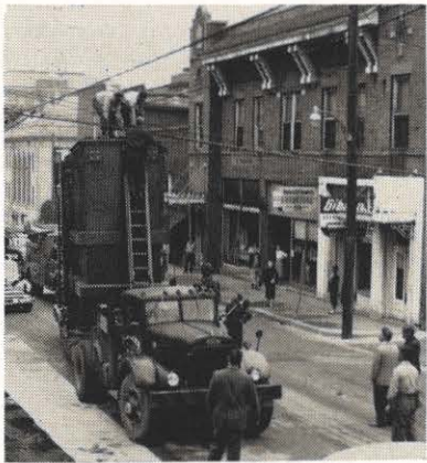
"Easy does it" is the by-word here. Telephone men in Marion were forced to hold up this main telephone line to permit passage of a giant transformer for the new Smythe station. Looking on at the right, wearing coats, are E. C. Rankin and J. S. Sutphin.
