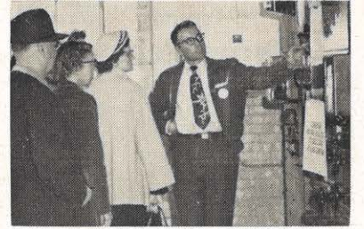
Vernon Greene, station foreman, explains the controls at Bellefonte substation to a group of the teachers.
