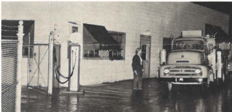
Following a 4 o'clock breakfast, crews load on trucks and get ready to leave the service building. Bud Syck, line foreman, is shown talking at left to Oscar Hamilton, line foreman, sitting in the truck.
