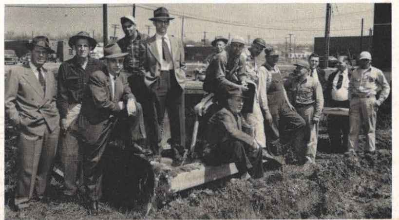
A group of Kingsport employees look over the site of the new service building as ground was broken on April 5. They are, from the left: J. E. Wright, vice president and general manager; L. E. Nutter, line supervisor; D. P. Blankenbeckler, stores supervisor; S. E. Russell, lineman; M. C. Simpson, commercial manager; J. A. Randall, meter supervisor; J. P. Smith, lineman; C. H. Hurd, truck driver-lineman; Lindsay Wade, lineman; Woodrow Ball, groundman; Hubert Greene, groundman; Clarence J. Bryan, assistant general manager; R. C. Scarlett, station supervisor; and J. J. Potts, working foreman.
