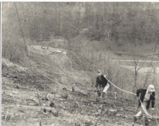
semi-circle) men are pulling the new conductor up the steep hill and into position. RIGHT: Pulling the heavy cable, the men climb on up, nearing the top.
