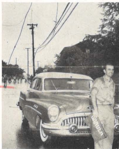
Severe electric storm in Beckley knocked out a main double circuit 44,000 volt line on South Fayette Street recently, blocking traffic for an hour and a half. Daniel E. Murray, lineman, is shown as he stopped traffic while other members of line crews in the background hastened to repair the lines. A driver of a trailer truck rendered aid to the company when he jacked up his truck in the middle of the road to help stop traffic for the linemen. There was also a failure in a Beckley substation transformer but service over the entire city was restored a little over three hours after the failure.
