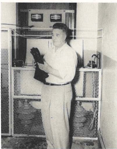
B. C. Currence, who has been testing gloves for 20 years in the Charleston division, removes a pair from the electric testing device. He will place them on a rack for a 24-hour drying period.
