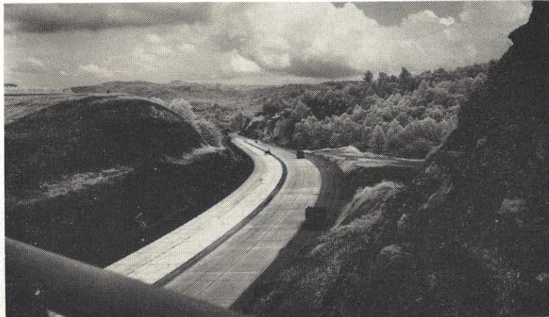
Section of four lanes in West Virginia Turnpike near Beckley shows the use of concrete creeper lanes for trucks. The highway has two 12-foot concrete traffic lanes throughout with these added lanes on grades to permit passing. Its three service areas, restaurant and service station facilities are located at Bluestone, Beckley and Morton. Interchanges are at Princeton, Beckley, Mossy, Chelyan, Kanawha City and Reed.
