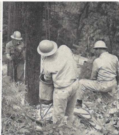
LEFT: Jess Collier and Ireland Layne hang blocks in preparation for the setting of a second pole in the structure. RIGHT: Red Clark, Ira Smith and Hylton Williamson busy themselves on the ground while the linemen above prepare for sending up of the winch line.
