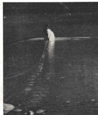
No, that's not a man on the wrong end of a fishing line. It's Jimmy Oliver, Hazard district line department employee, carrying out another of the varied duties of a lineman. During construction of a rural line extension, employees found that there were no boats or bridges to help in carrying the line across the Kentucky River. So Jimmy gamely shucked his clothes and started wading and dragging. A couple of times he thought he might have to swim but he got that line across.
