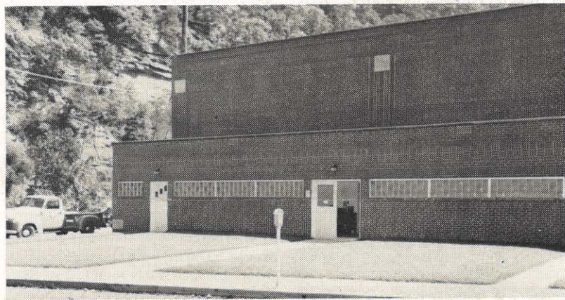
Whitesville area office in the Charleston district moved into these new quarters recently. The new building provides modern offices for the accounting department, service and meter supplies and appliance repair shop. Future plans call for installation of an all-electric kitchen and appliance demonstration facilities in the building's 42 by 32 foot auditorium.
