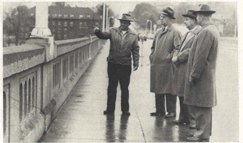
Inspecting the new lighting on Rivermont Bridge in Lynchburg are, from the left: R. H. Porter, working foreman, in charge of installing the fixtures; D. C. Kennedy, district manager; J. R. Martin, line and station supervisor; and P. L. Bailey, district superintendent.
