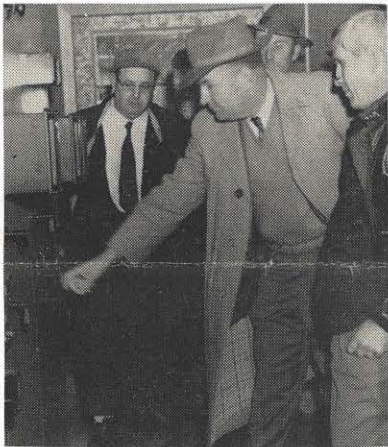
Additional source of power for the Lynchburg area was provided when P. L. Bailey threw the switch that energized the new South Lynchburg station December 9. Looking on are, from the left: J. J. Armstrong, system operating supervisor; E. C. Rankin (face partly hidden), supervising substation engineer; Ted Carroll, system relay engineer, and R. L. Hatch, Reusens hydro plant supervisor.
