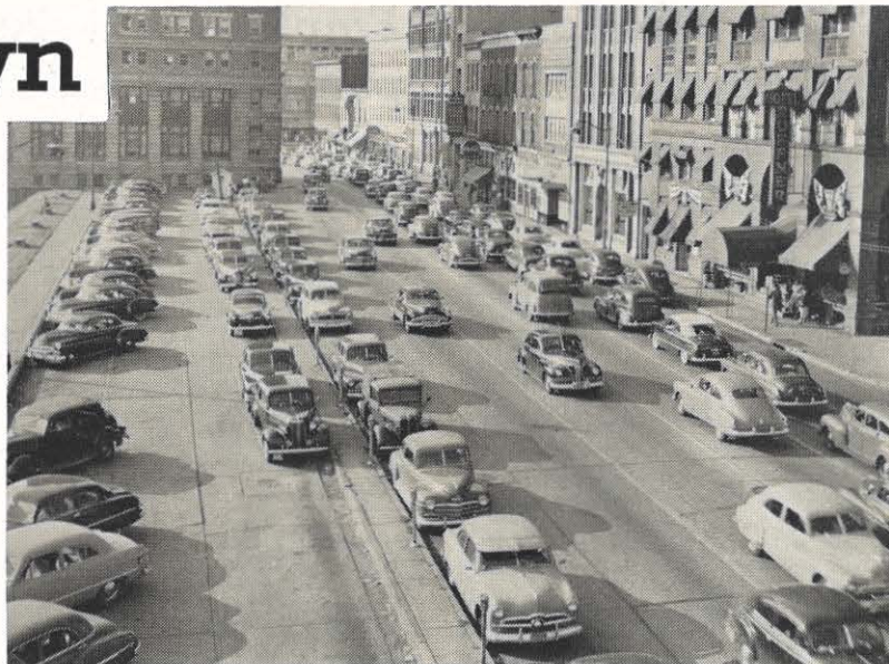
The need for modernizing today's roads is upon us . . . even without our new millions of babies. Kanawha Boulevard in Charleston is an example of meeting the needs of roads which are carrying 55 million vehicles, 72% more than in 1940.
