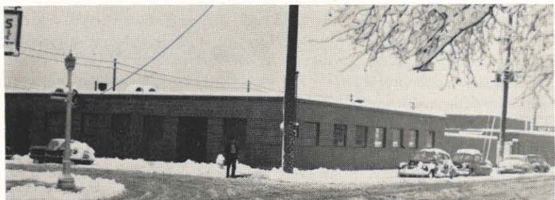
Kingsport's recent snow found crews working out of the new Cumberland service building which was occupied January 3. Cumberland distribution station is located in the rear.
