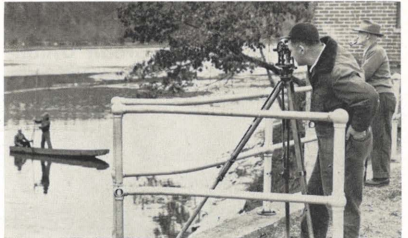
Actions of these Pulaski district employees bring back memories of the steamboat days of the old South. G. B. Chumbley, seated, and D. B. Smith are sounding for mud depth at the Byllesby dam while G. P. Williams takes the reading. All three are instrumentmen. King Mustard, Byllesby plant foreman, looks on. Sounding for mud depth so that eventually the mud can be removed to make way for more water is similar to the sounding done from the decks of the old steamboats. Steamboat men used lead weighted strings while these modern day sounders use a pole, but both groups shouted their findings to a recorder.
