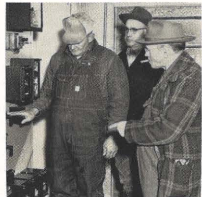
Checking switching procedure at the control panel at Smyth station are, from left, C. B. Sharpe, W. B. McGlothlin and J. S. Sutphin.
