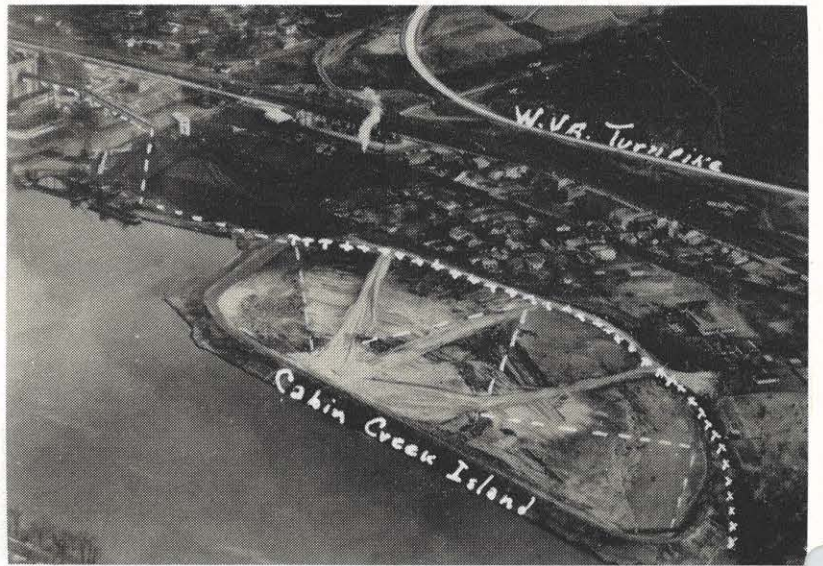
Showing the fly ash disposal area for Cabin Creek plant, the dotted line is the flow of fly ash from the plant's new dust collectors. Fly ash is sluiced from the plant by pipe line and enters the basin at the upper left area near the coal storage yard. Three earthen dikes, the fourth under construction, form settling basins for the dust particles. The x-mark line shows where the channel which formerly separated the island from the mainland was filled in.
