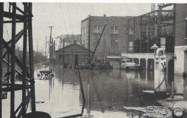
Williamson service building was flooded for the first time since it was built in 1928. Water depth in these buildings varied from 2 to 4 feet. Material had to be removed from these buildings.
