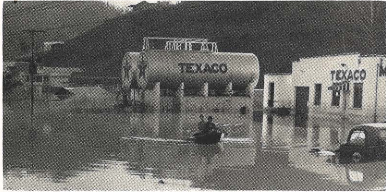
Heading for shore after replacing a customer's meter are Ottis Blankenship and Harry Trimble, meter department employees in Paintsville of the Pikeville district. Note house in background with only roof above water.
