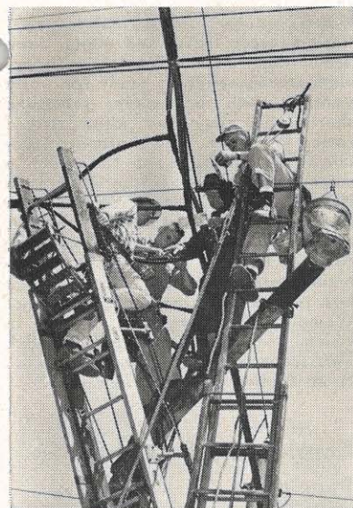
H. L. Back guides the spinner as it lashes power lines together with plastic lines. Photo courtesy 'Huntington Advertiser.'
