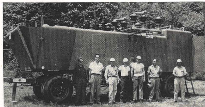
The Logan station crew line up after the new 3,000 kva mobile substation was put in service for the first time. The 20-ton station is the first to be used in the district. Shown from the left: M. M. Donohoe, Howard Fogleson, Paul Adams, Jimmy Sullivan, Dallas Kinser, G. A. Blankenbeckler and A. C. "Jack" Fife, station foreman. The men recently energized the station for the first time and were able to provide continuous service to customers while major maintenance was being done at Becco station, a vital central switching point. The station also to be used for emergency replacements in case of failure of transformers or other major equipment, will also serve Williamson district.
