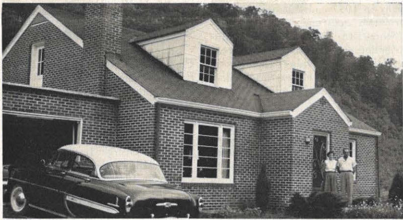
Mr. and Mrs. Lewis York stand before their seven-room home that took them five years to build on the "pay as you build plan." Their home near Hazard is debt-free.
